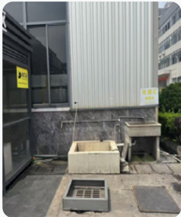
Floor Washing Water Three-Stage Sedimentation Tank
